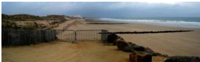
Figure 3. Groins (from the top of the riprap of Les Becs to the south).
