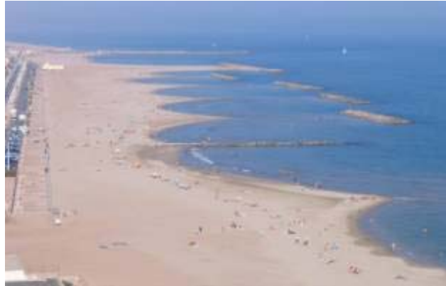
Figure 3. Coastal structures (constructions and protection works) at Valras (Hérault, France): jetty, detached breakwaters and a groyne made of rock (from the background forwards) (© CETMEF).
