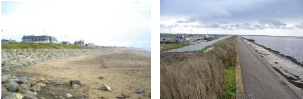
Figure 2. Examples of shore-parallel defences: rock-revetted seawall at Barneville (Calvados, France, left) and revetted dike at Beauvoir-sur-mer (Vendée, France, right) (© CETMEF).
