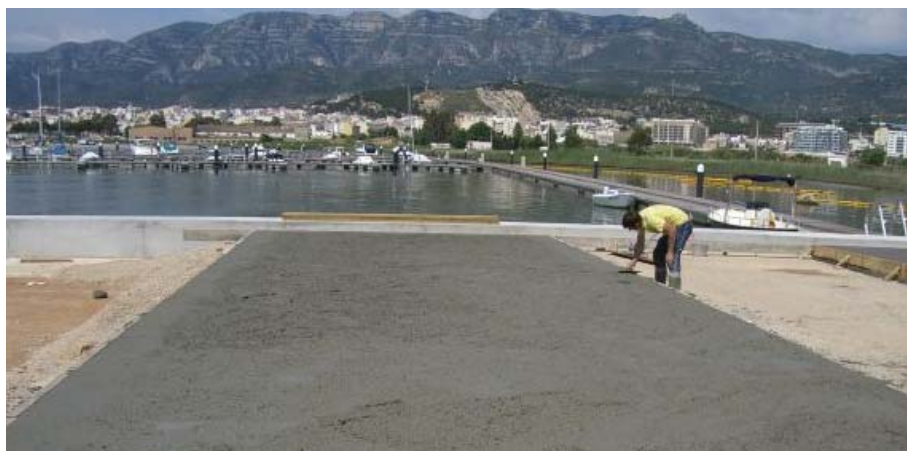
Figure 1. Pavement execution, after LIMEIRA (2011).
