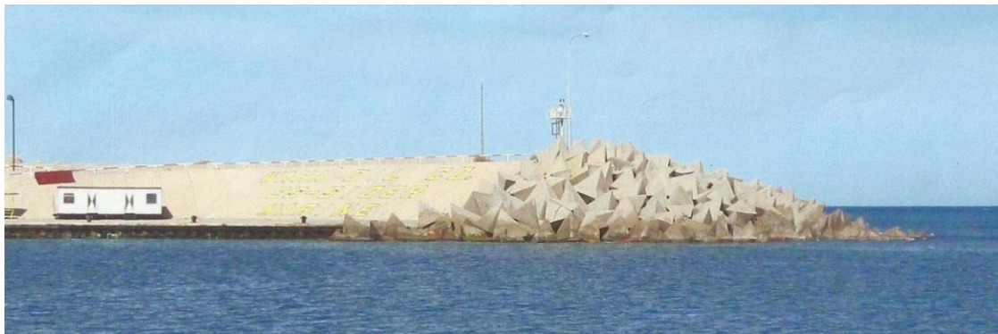
Figure 3. Photo of the breakwater, including the section at the head (16/02/2011).
