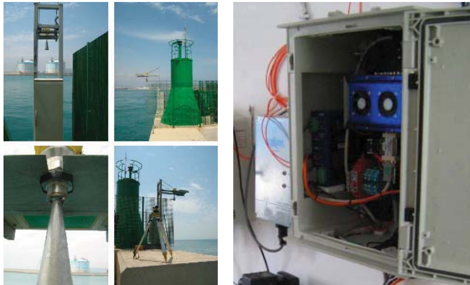
Figure 1. MIROS Range Finder station in Sagunto Port. The sensor is tested for right operation by comparing its measurements with a Vega Puls 62 (radar technology). Data is stored in an embedded PC and transmitted through GPRS.
