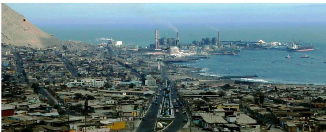
Figure 2. El Salitre beach and port region before the construction work.
