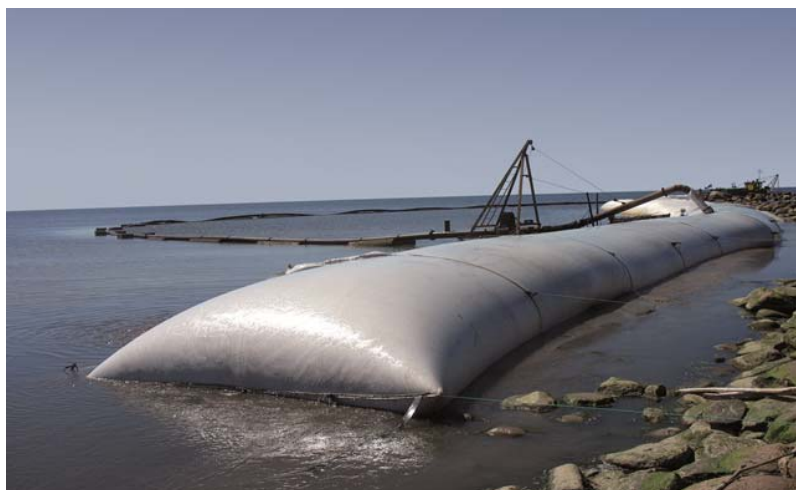
Figure 1. Geotextile tube used for coastal protection.
