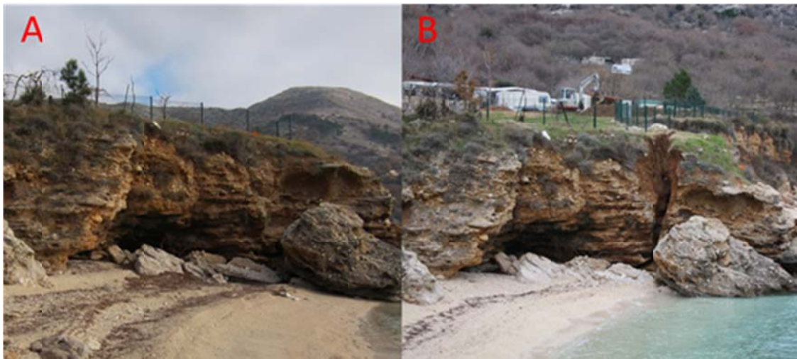
Figure 2. Before (A) and after (B) the collapse of a cliff near Stara Baška, (February 2014).
